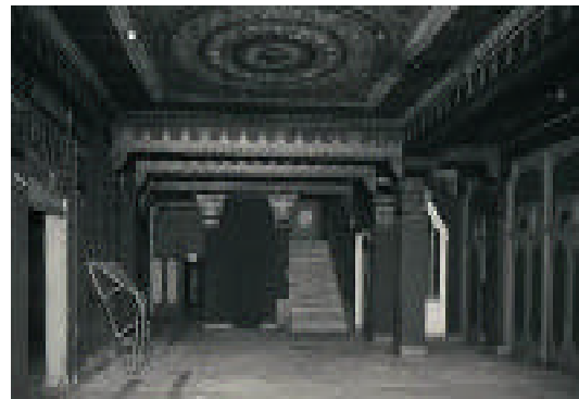
Figure 17: Main floor foyer
