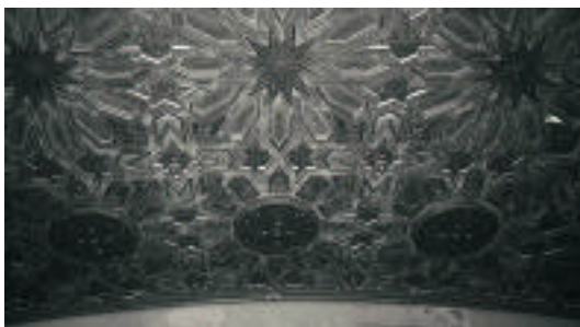
Figure 14: Auditorium ceiling at the rear wall
